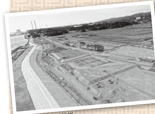
復旧が進む前原の沿岸
